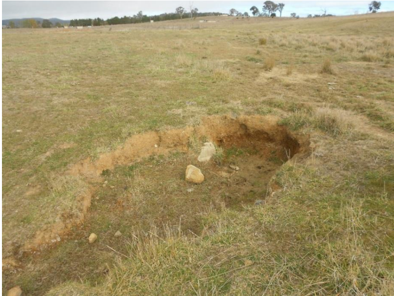
Figure 24: Eroding overflow of Dam 3.
