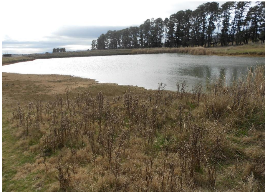
Figure 21: Dam 5 showing signs of saline discharge in and around top water level.
