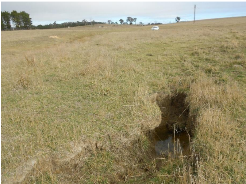
Figure 25: Eroding overflow of Dam 3.
